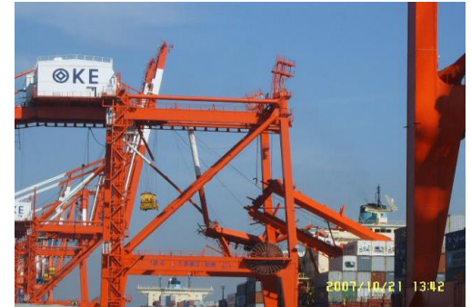
Crane Collapse Korea
